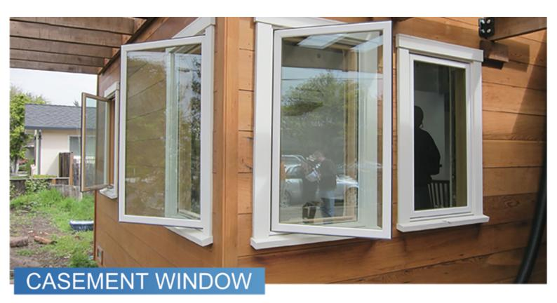
Created to allow more ventilation into your home, the Superhouse casement window captures the essence and tradition of the past. Combined with the design versatility and slim appearance of aluminum, the casement window is ideal for locations where you want to maximise the view with large unobstructed areas of glass.
