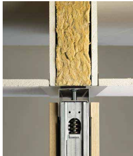
Ceiling element with steel panel and insulation
