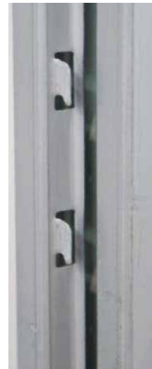
Hook structure on wall panels allows easy set-up
